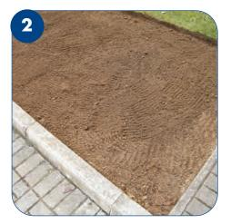
Prepare ground and make level. Put down a layer of Type 1, 15 cm deep.
