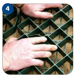
Clip tiles together, allowing for any cut sections to be the furthest away from heavily trafficked areas.
